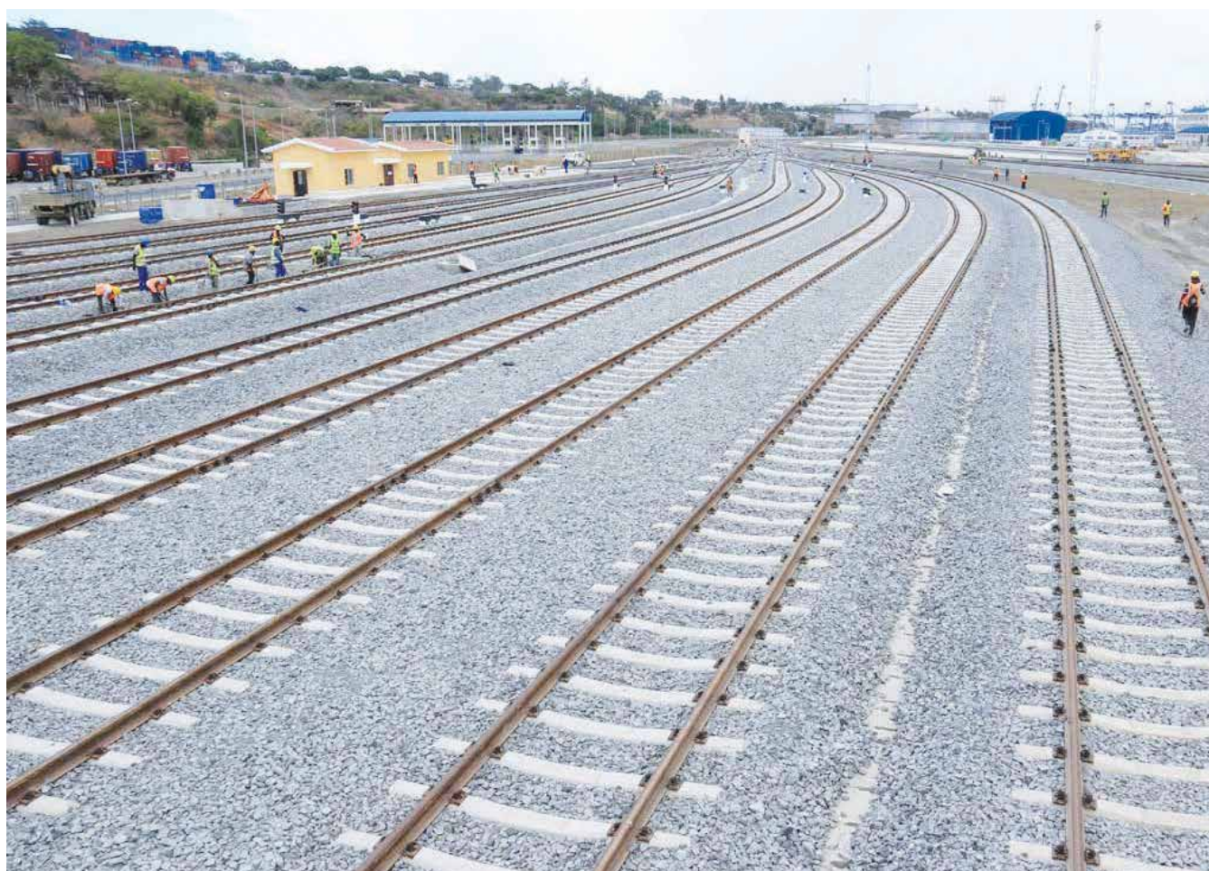
SGR Construction going on
