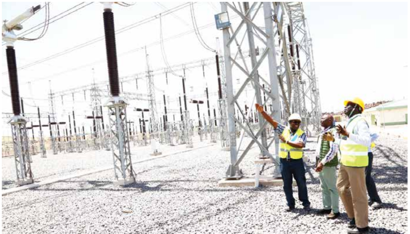
Loyangalani Transmission Line
