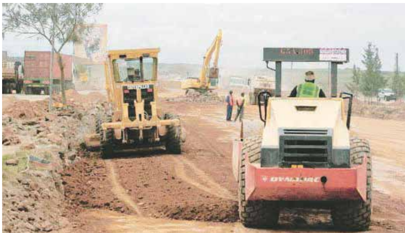
Eldoret-Turkana road under construction
