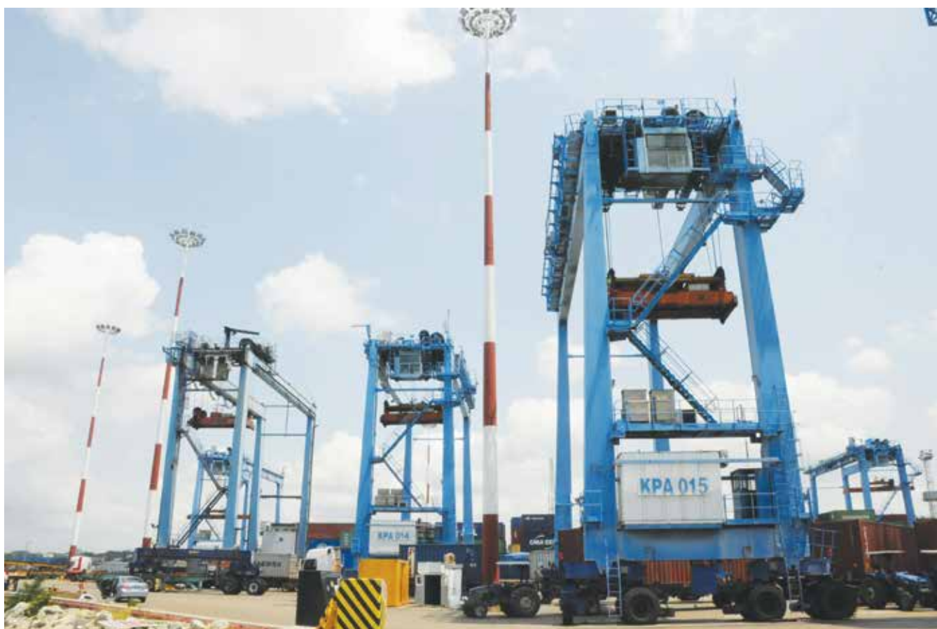
Mombasa Port Berths
