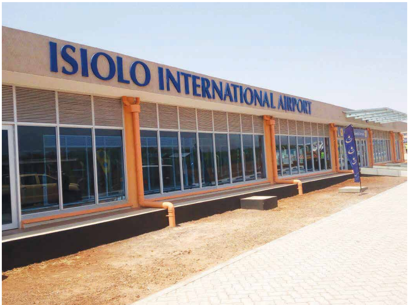
Isiolo International Airport under construction
