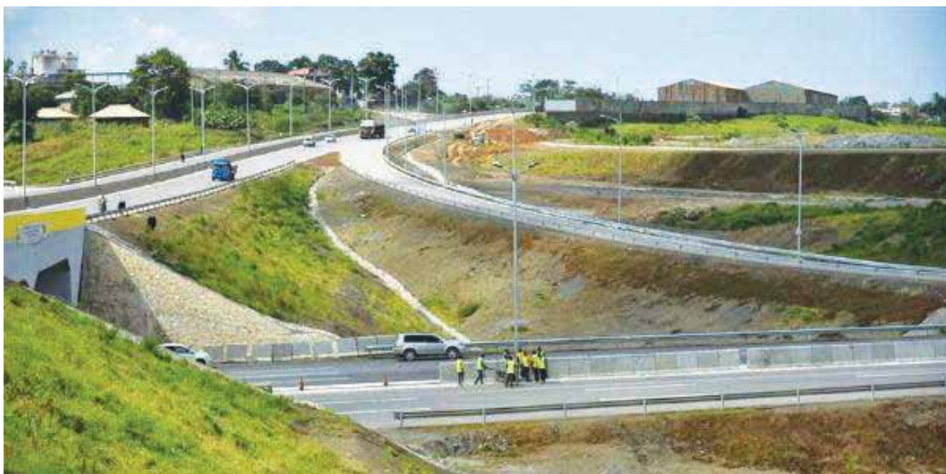
Recently completed section of Dongo Kundu Road, Mombasa
