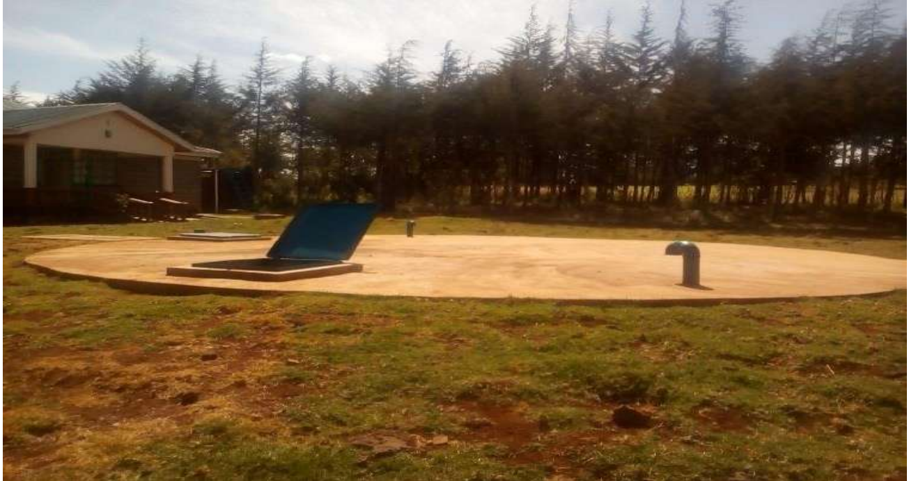
Figure 2: Underground Water Tank
