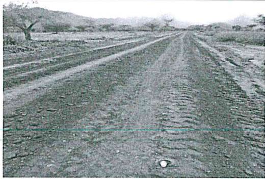
Figure 1: Kacheliba-Nakwapuo-Cherangan road grading
