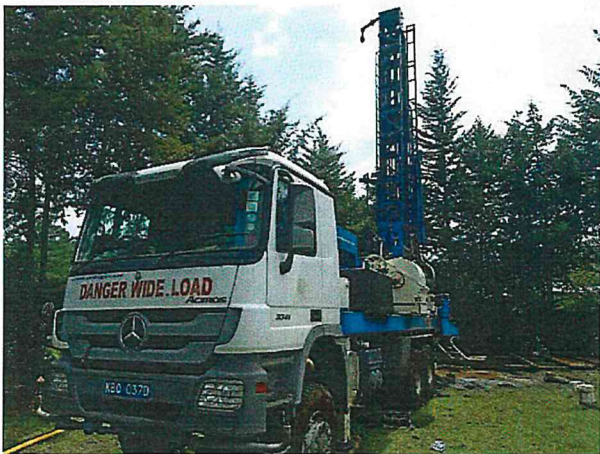
Drilling Community boreholes in Nyandarua County
