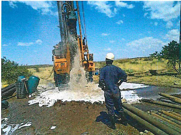
Drilling borehole at Tullu Roba Mosque Compound Isiolo County
