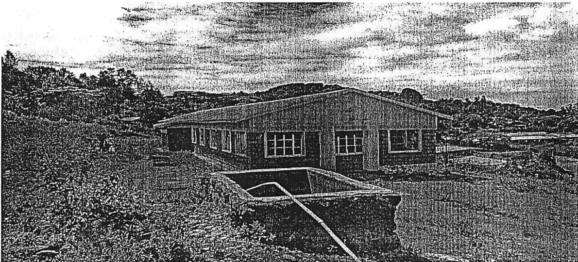
Kipsaraman D. O's Office – Construction of Offices
