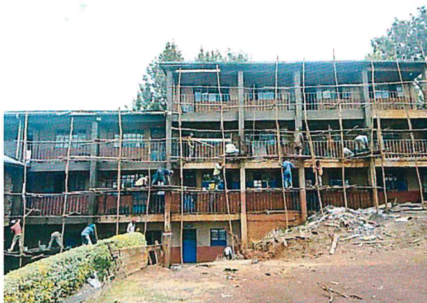
Plastering columns & beams externally on going
