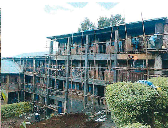
Plastering columns & beams externally on going
