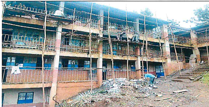
External plastering on columns and beams.
