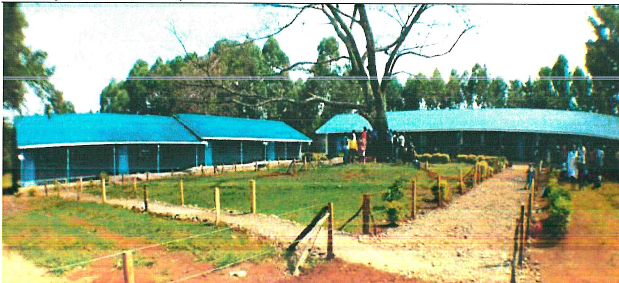
Fig 3: Ringa Primary School: Rehabilitation of 14 Classrooms
