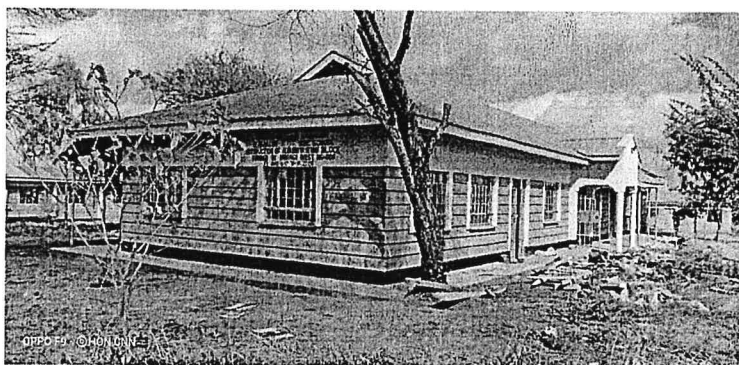
FIG 1.2: Administration block constructed at Kavaini Secondary School, completed FY 2019/2020 to improve teaching staff welfare.
