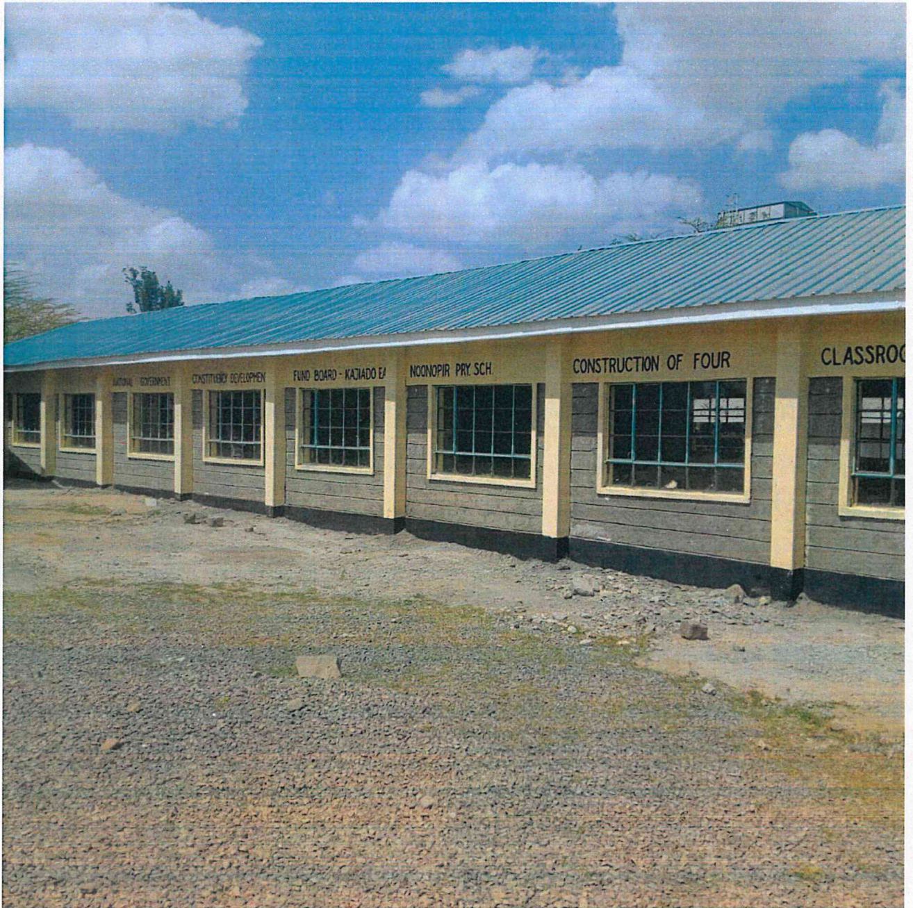
Noonkopir primary school construction of 4 classrooms.
