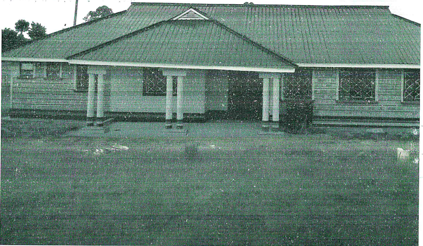
KWANZA OCPD, CONSTRUCTION OF OCPD'S OFFICE-COMLETE.
