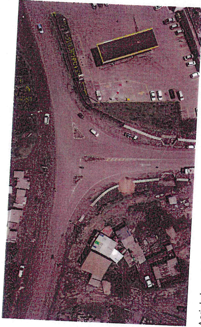
New 32m long two span concrete bridge at KM 35+346 along Kajjado – Imaroro project corridor
