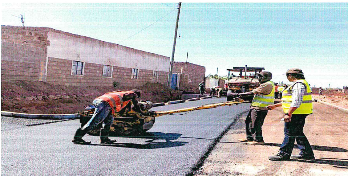
Construction of Kajiado Town Roads Phase I
