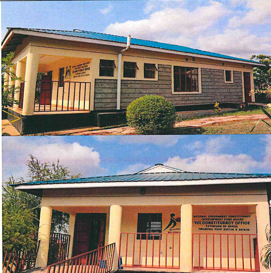
EXTENSION OF NG-CDF VOI OFFICE
