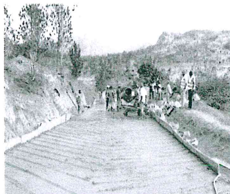
Expansion, grading and slabbing of Kese –Mzazala-Saghasa road in Werugha Ward, Wundanyi sub-county.
