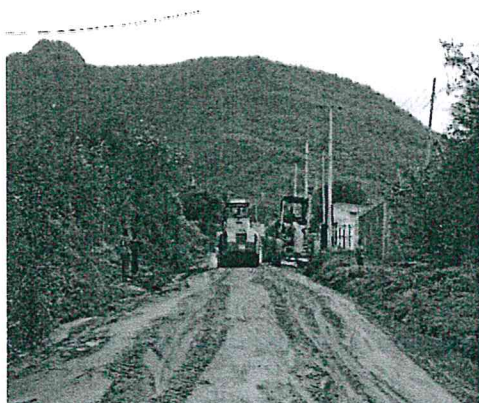
Murraming of Kaloleni feeder roads in Voi.
