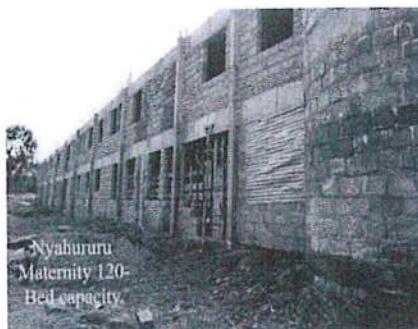
Underway Nyahururu's 120 bed capacity maternity facility.
