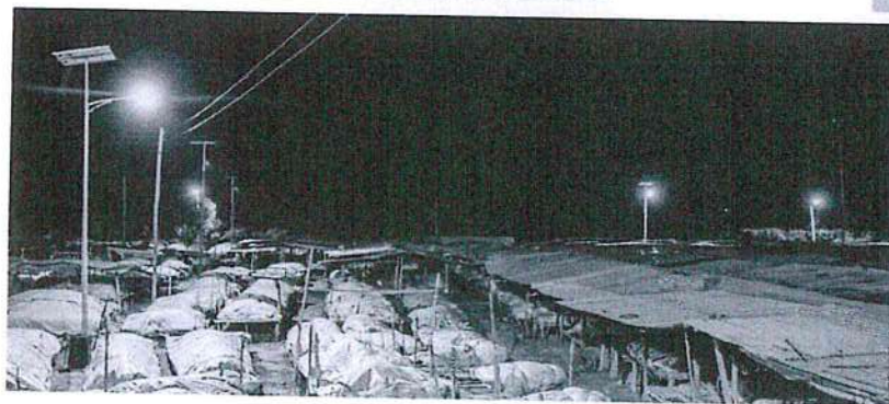
Nanyuki Market lighting- one of the initiatives aiming to boost efforts to have 24-hour businesses.
