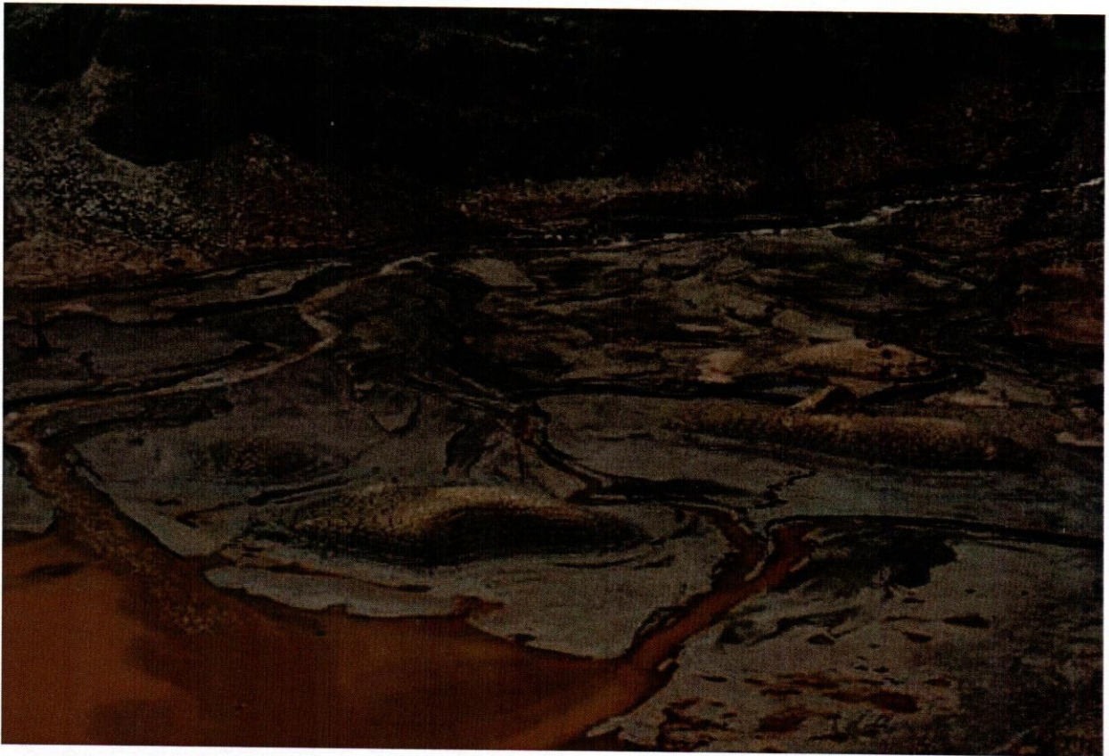
Tunderess River flowing into the Tunderess Dam, the dam was drained following the collapse of the Milmet Dam. (Picture taken on 6 th July 2018)
