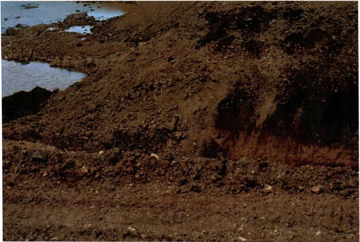
Section of the Milmet Dam that was unblocked to release water to flow downstream ( Picture taken on 6 th July 2018 )
