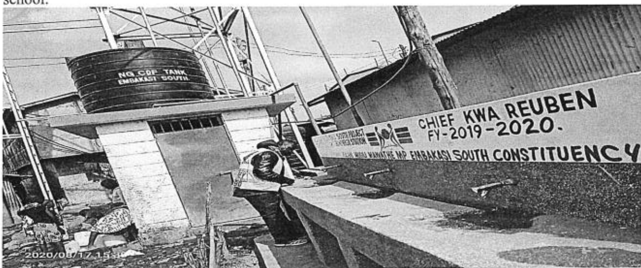
FIG 1.1 Kwa Reuben Chiefs Camp construction of Hand Washing Stations.
