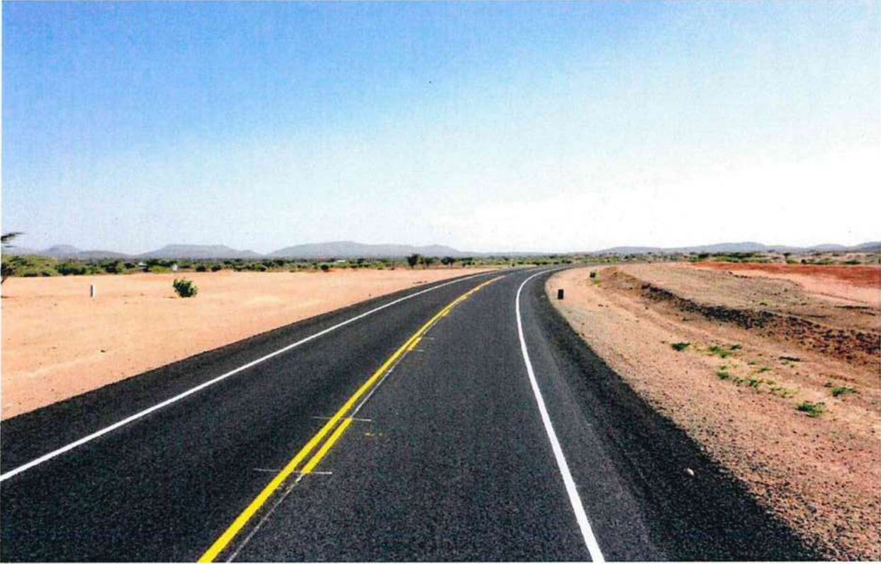
A section of the Lokichar-Lodwar-Nakodoko 330 Km Highway
