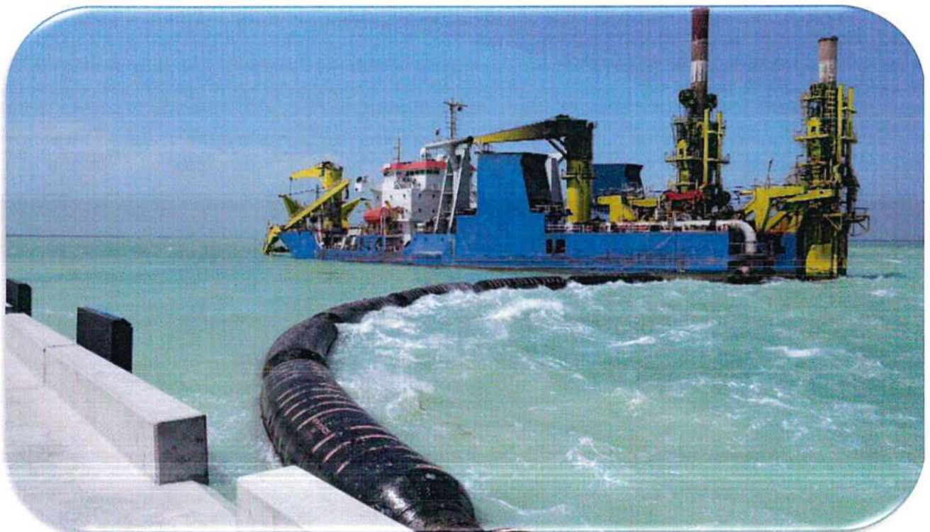
Figure 2: Dredging channels at the Port of Lamu
