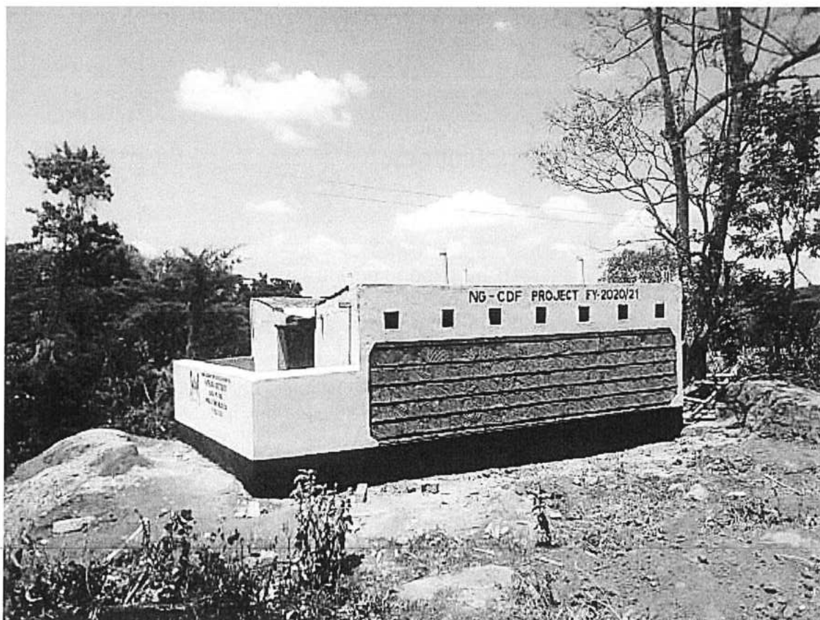
NASOKOL PRIMARY SCHOOL TEN DOOR TOILETS
