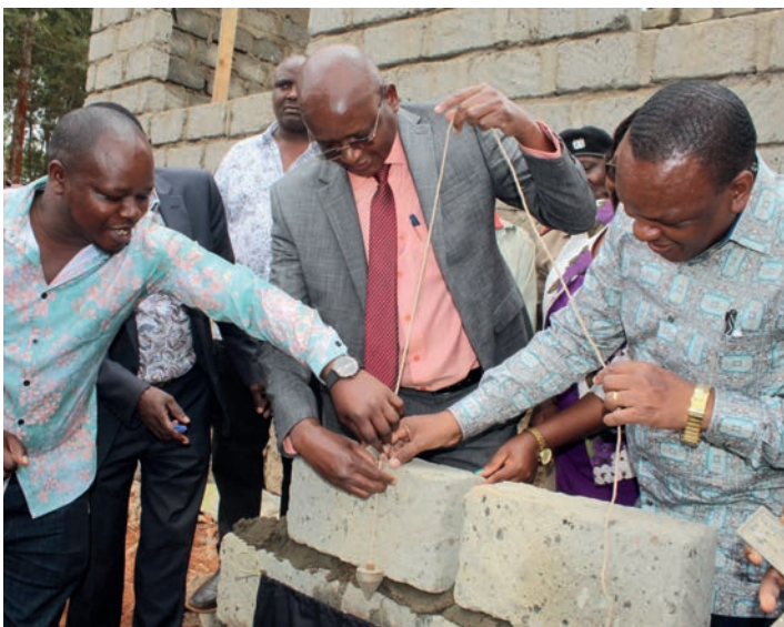
K aiti MP, Hon. Joshua Kimilu (in floral shirt) accompanied by the National Government Constituencies Development Fund Board Chief Executive Officer, Mr. Yusuf Mbuno and the Constituency CDF staff launch the construction and equipping of an administration block at St.
