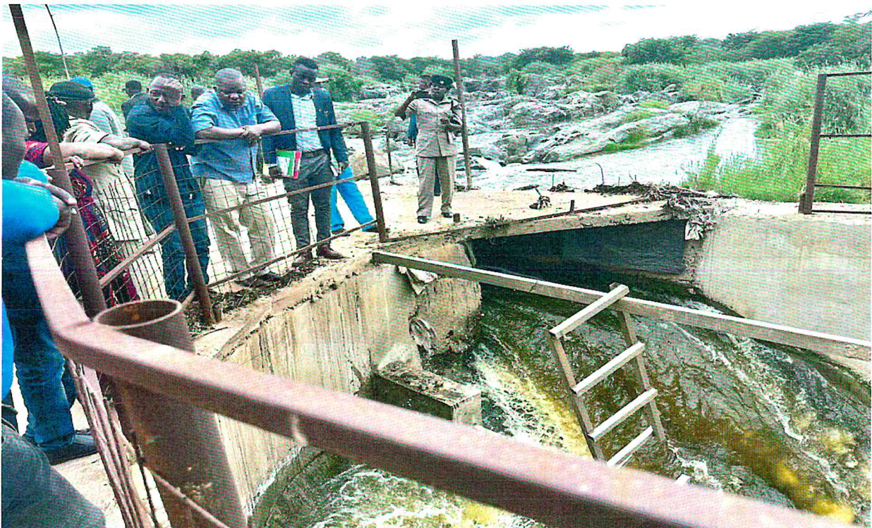
Figure 8. Members of the Public Petitions Committee inspecting the dam project along River Athi, at Kiukuuni Village in Mwala Constituency
